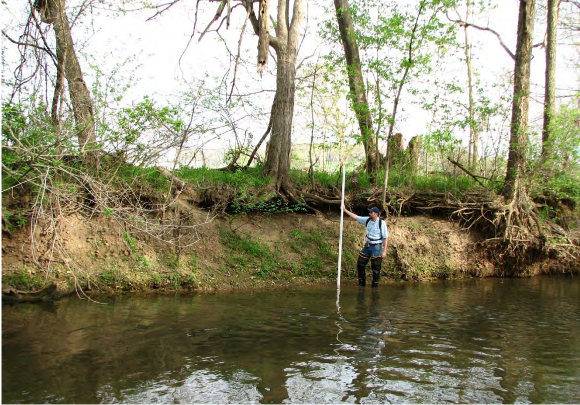
Photo 13 – Moderate streambank instability that would be addressed at Area 2
