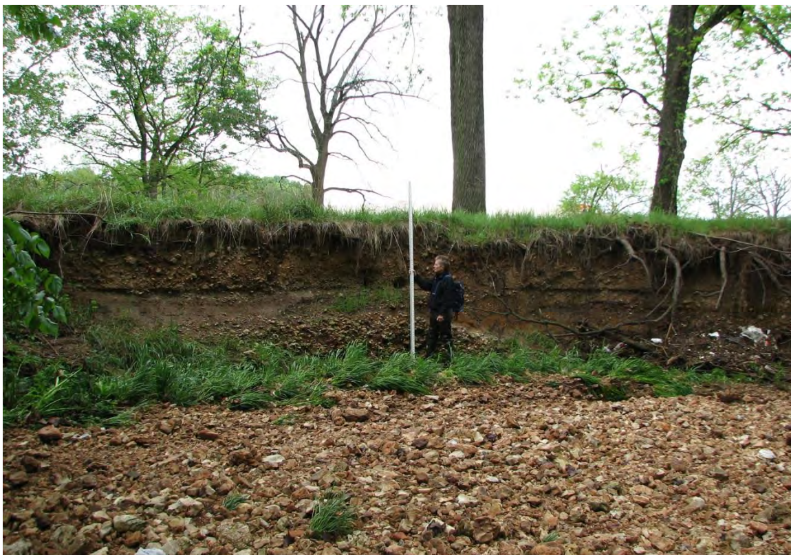
Photo 21 – Incised stream channel with bankfull scour lines
