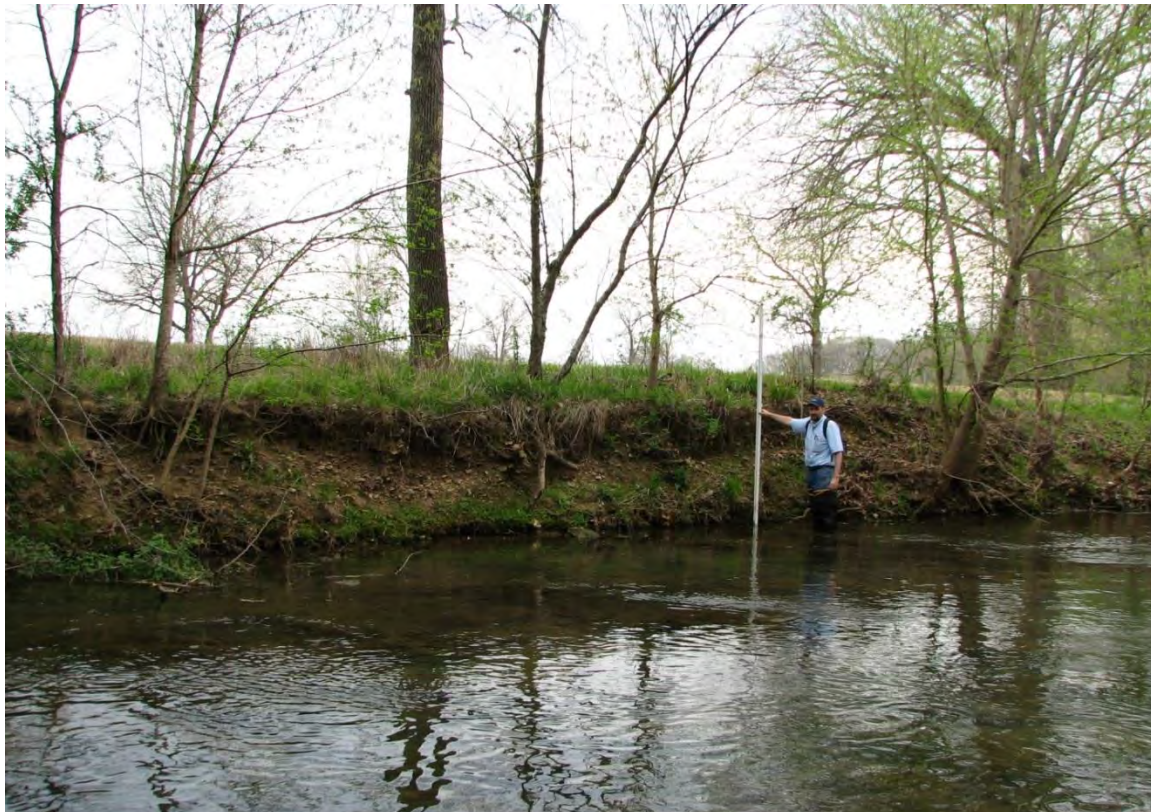
Photo 11 – Eroding streambank in Area 2 that will be restored
