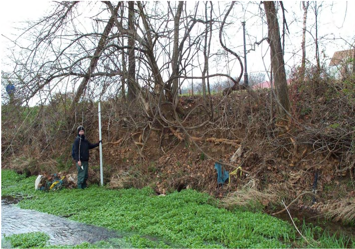
Photo 21 – Eroding streambank and riparian in Area 3A that will be restored
