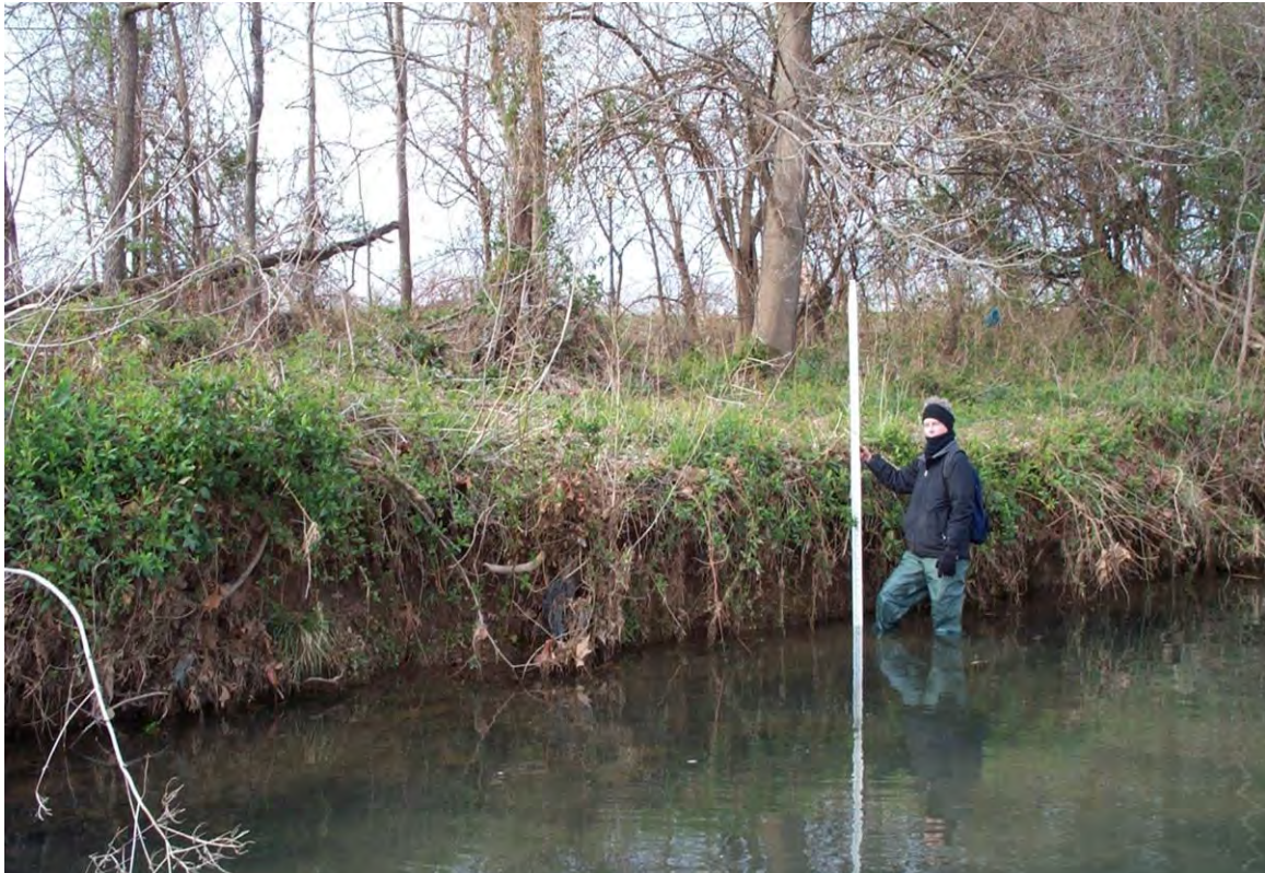
Photo 20 – Eroding streambank in Area 3A that will be restored
