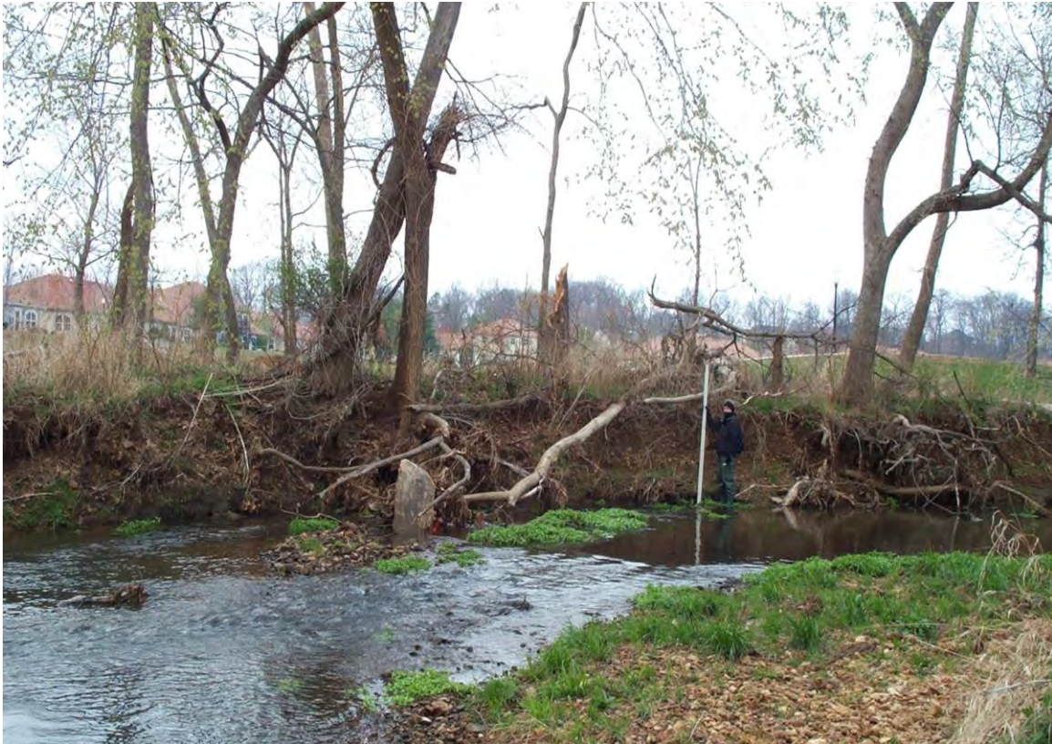
Photo 19 – Eroding streambank in Area 3A that will be restored
